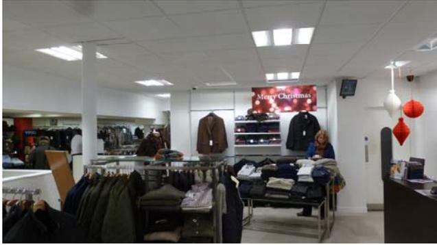
Menswear used the Gullwing LED and Standard LED Asymmetric KLRA and the Toy Store used the same with the addition of a specially developed Swingline fitting. This area had low ceiling with no void and these surface 3 directional fittings work really well giving plenty of light and creating an interest to draw people from the door towards to rear of the store. Thames Downlights were also used in areas where the Gullwings could not be installed.
